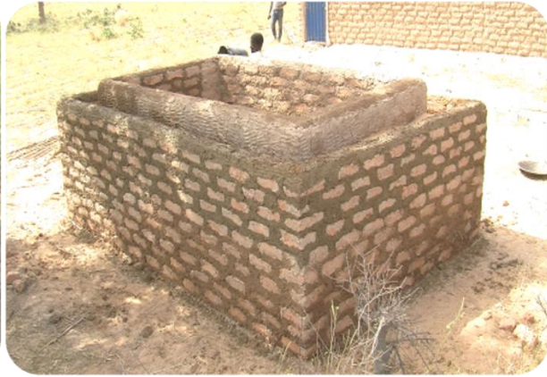
Zero Energy Cooling Chamber
