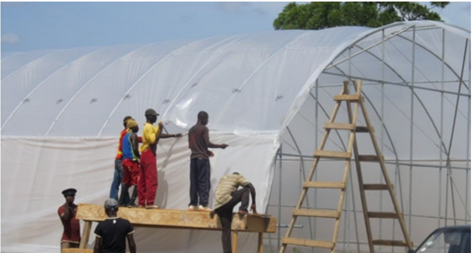
Tunnel greenhouse being built in Ghana.
