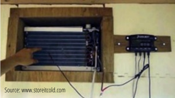
An air conditioner with a CoolBot unit connected to its controls.
